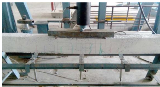
Figure 7. Flexural cracks at Ultimate Load
