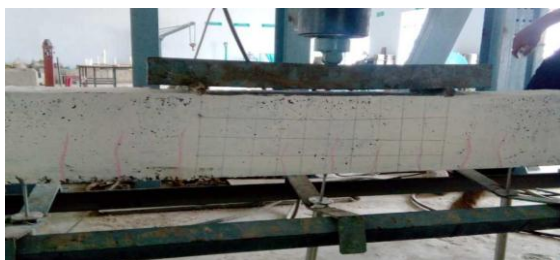
Figure 7. Initial Crack pattern
