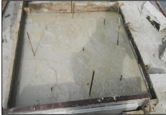
Figure 7. Slab with steel fiber
