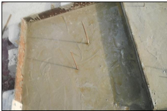
Figure 7. Slab without steel fiber
