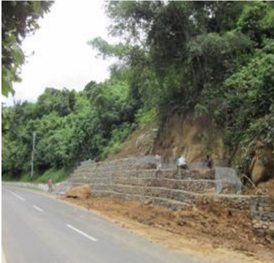
**Figure 7** Remedial action using gabions
