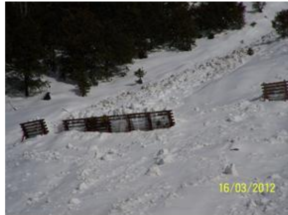
Figure 9 Winter view of snow bridges at experimental site
