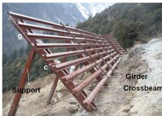
Figure 1 Overhang of crossbeam 'c' & girder 'g' and internal angle of support 'φ'
