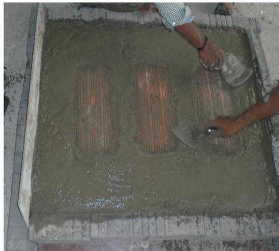
**Fig-5** Showing the casting of the Concrete slabs
