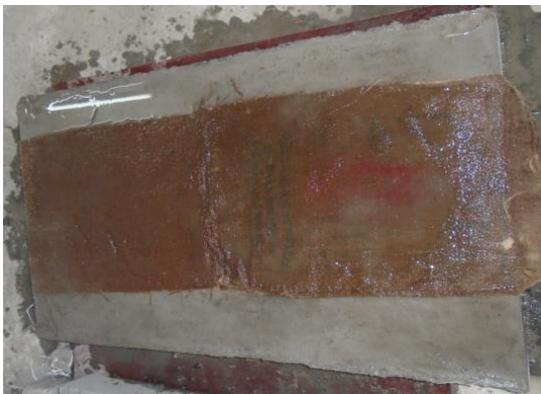
**Fig 7** Showing the curing of the slab
