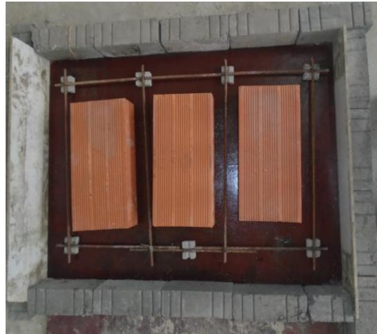
**Fig-4** Showing the placement of the porotherm blocks and the steel bars.
