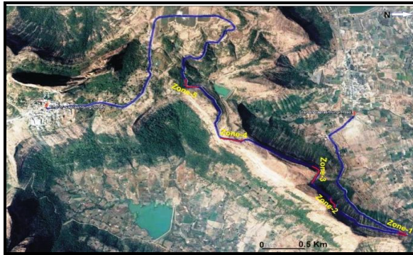
Figure 1 SGT curve road shown by blue line and location of rockfall prone zone marked by red line.
